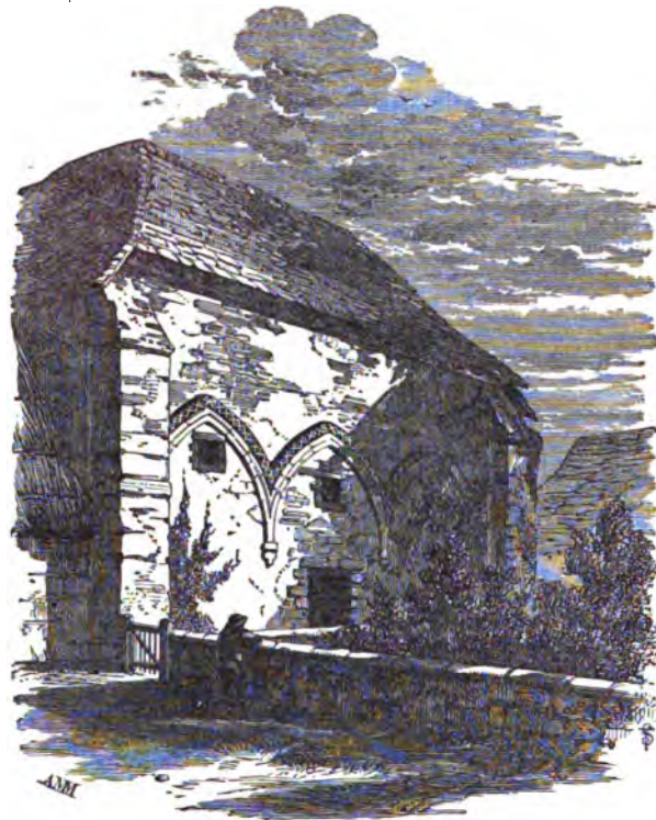
EXTERNAL VIEW OF THE EAST END OF HARDHAM PRIORY CHAPEL.
